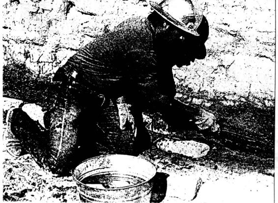
Coving—the bollowing out of an adobe wall just above grade—may be caused by standing rainwater, rainwater splash-up from the ground, or by salts deposited in the adobe by moisture evaporation. This adobe wall is being patched in the traditional manner with adobe mud.
