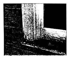
Deterioration of poorly maintained windows usually begins on horizontal surfaces where water collects. Problem areas on this sill are clearly indicated by paint fallow due to moistine.
