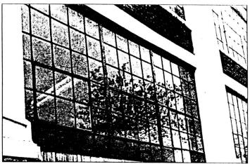
The steel pivot windows in this historic manufacturing building were replaced with new windows which matched the multilighted originals.
