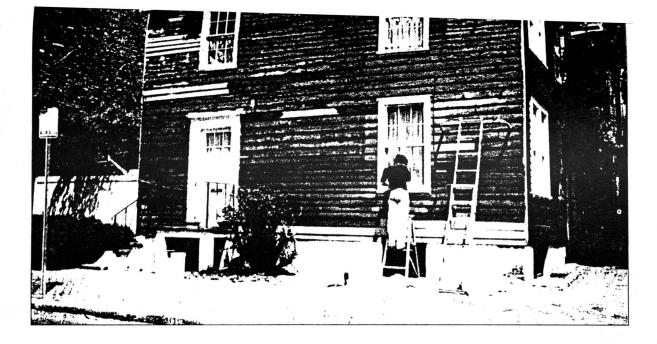
Using with care electric hot-air guns on decorative wood features and electric heat plates on flat wood surfaces when paint is so deteriorated that total removal is necessary prior to repainting.
