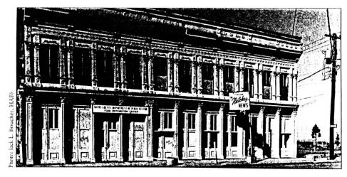
Deteriorated portions of the decorative pressed metal cornice have been inappropriately replaced with nonmatching, plain metal sheets, adversely affecting the historic character of this building.
