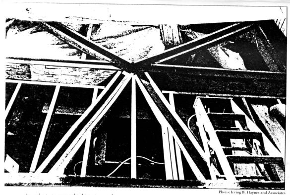
broider to preserve this historic woodpane building, new steel framing was in ted to reinforce the wood post and Lean structure. Original wood framing menders were notched to accommodate if e new steel frame.
