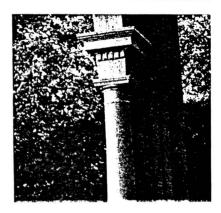
To replace deteriorated portions of the column, strips of new wood were milled to conform to the shape and appearance of the old column framework, glued in place, then back-primed and painted.
