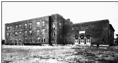
Councill (Negro) Elementary School (1926, 1928) 1400 Avenue M, Ensley
