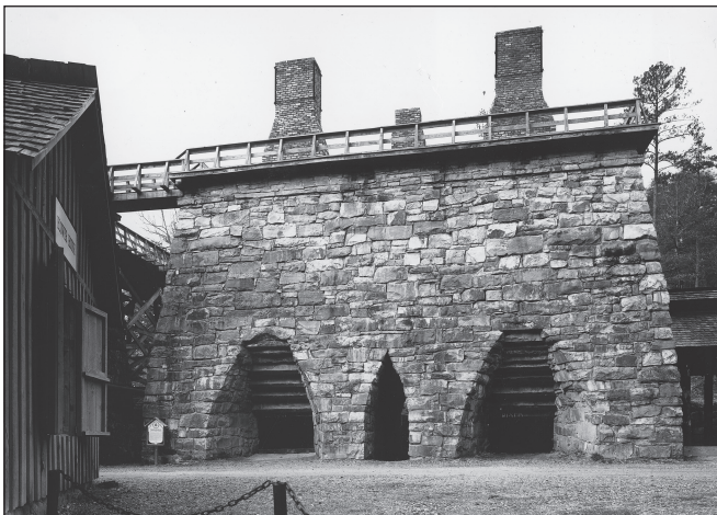
Tannehill Furnaces Nos. 1 and 2. Photograph by Jet Lowe, 1993. HAER AL No. 126.
