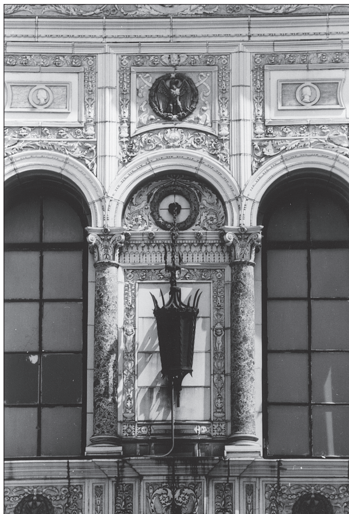
Terra cotta and marble detail, the Florentine Building. Photograph by Richard W. Sprague, Birmingham Historical Society, 1977.
