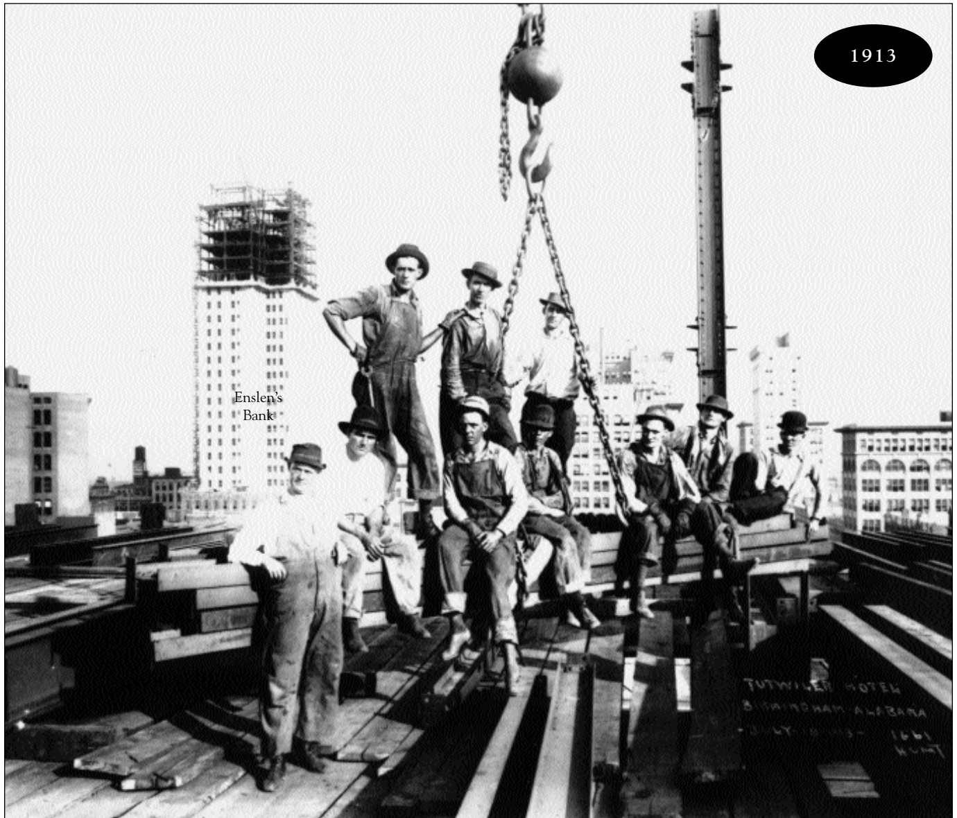
Construction crew at the old Tutwiler Hotel on 20th Street
