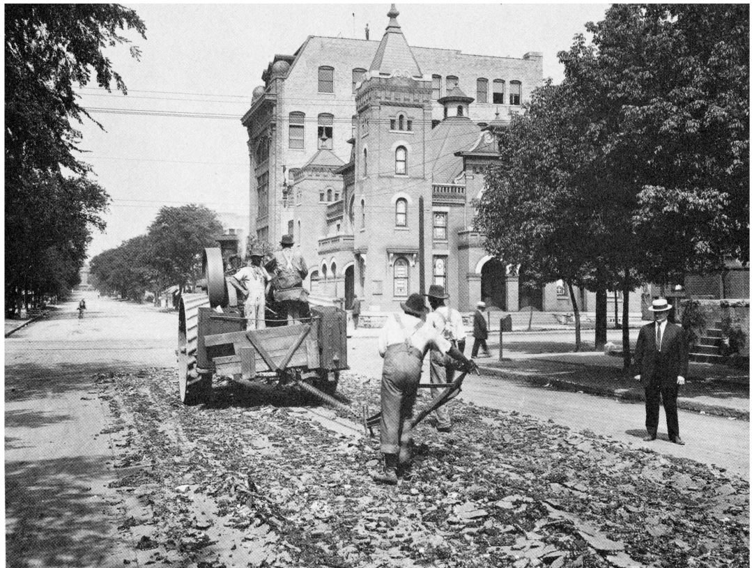
The scene is 5th Avenue and 21st Street North in 1912, and the street is being plowed up in preparation for the tracks of the Tidewater Carline. On the corner to the right of the workers is the First Christian Church and next to it is the Age-Herald Building; the Redmont Hotel now stands on this corner.
