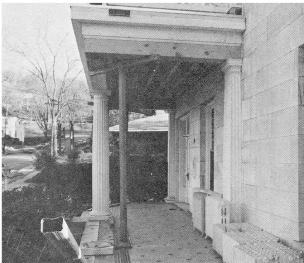
Reconstruction of exterior columns. Photograph courtesy Steve Trimmier and Bob Carney.
