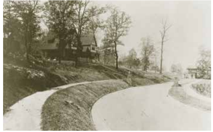
Dimmick House at the Cliff Road entrance to Mountain Terrace. Bert G. Covell, 1910. BPL Archives.
