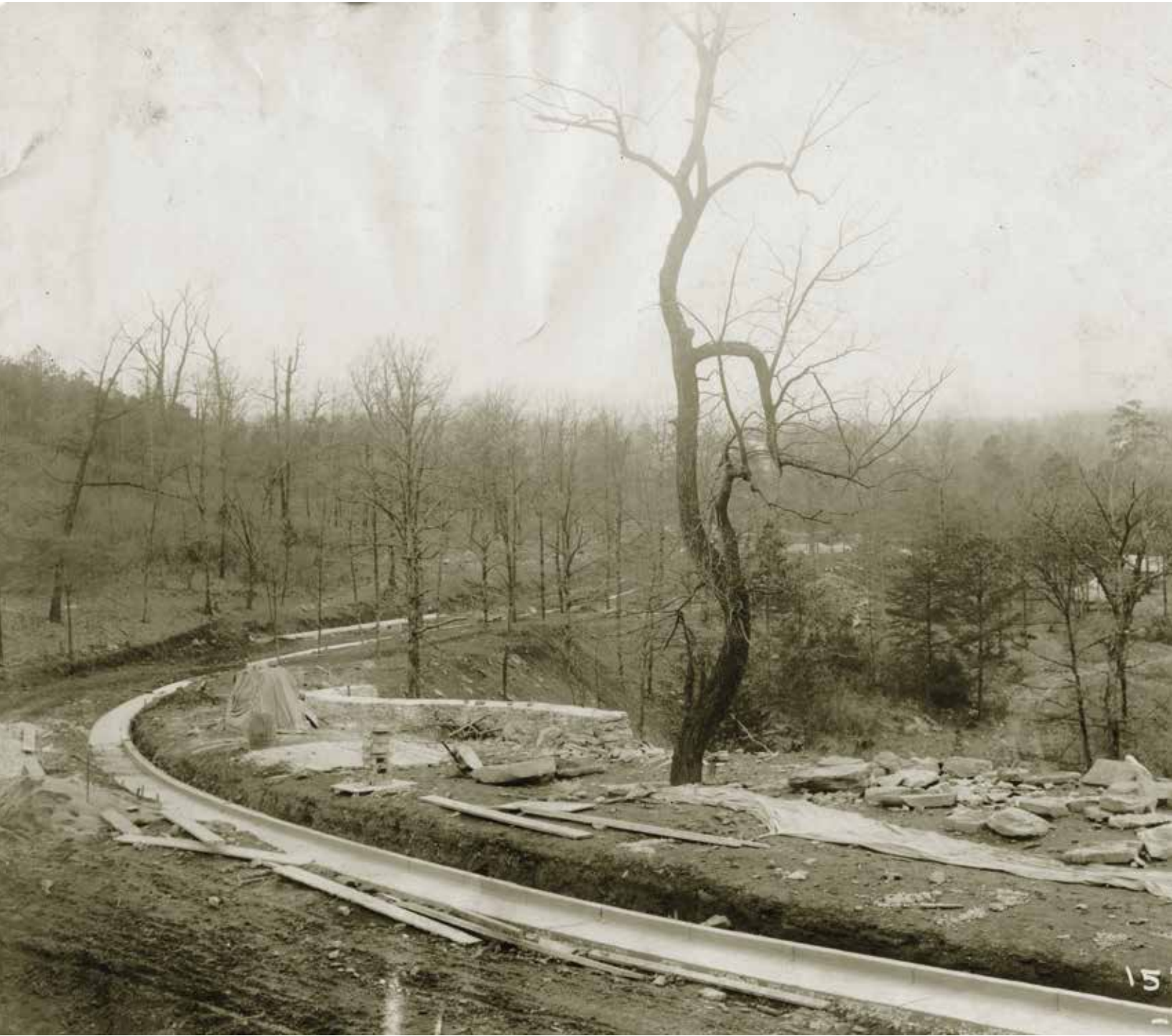
Cliff Road extension to Altamont, Glenwood, with retaining wall above the quarry, center, 1913. BPL Archives.
