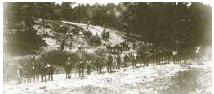
Road construction crew , grading to produce a smooth road. BPL Archives.
