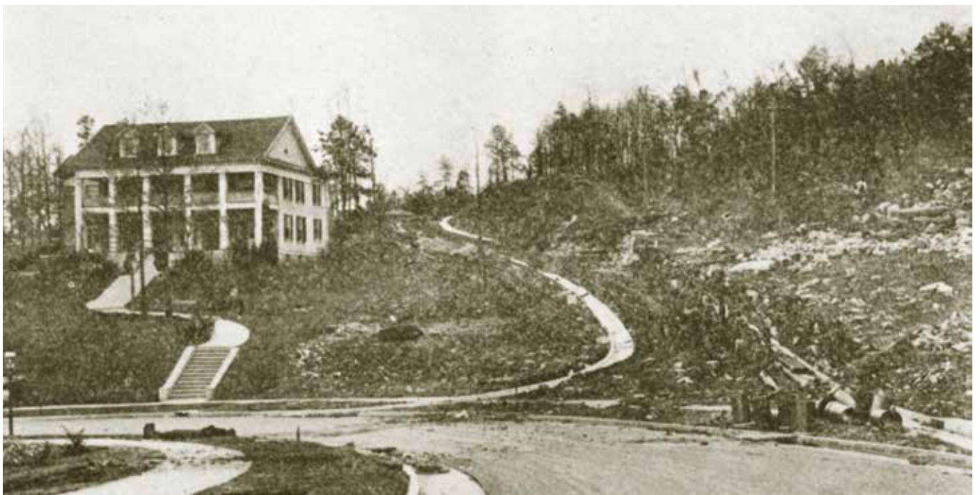
At work building Cliff Road , up to Glenwood, with the Ferguson House, on the left , 1913. BPL Archives.
