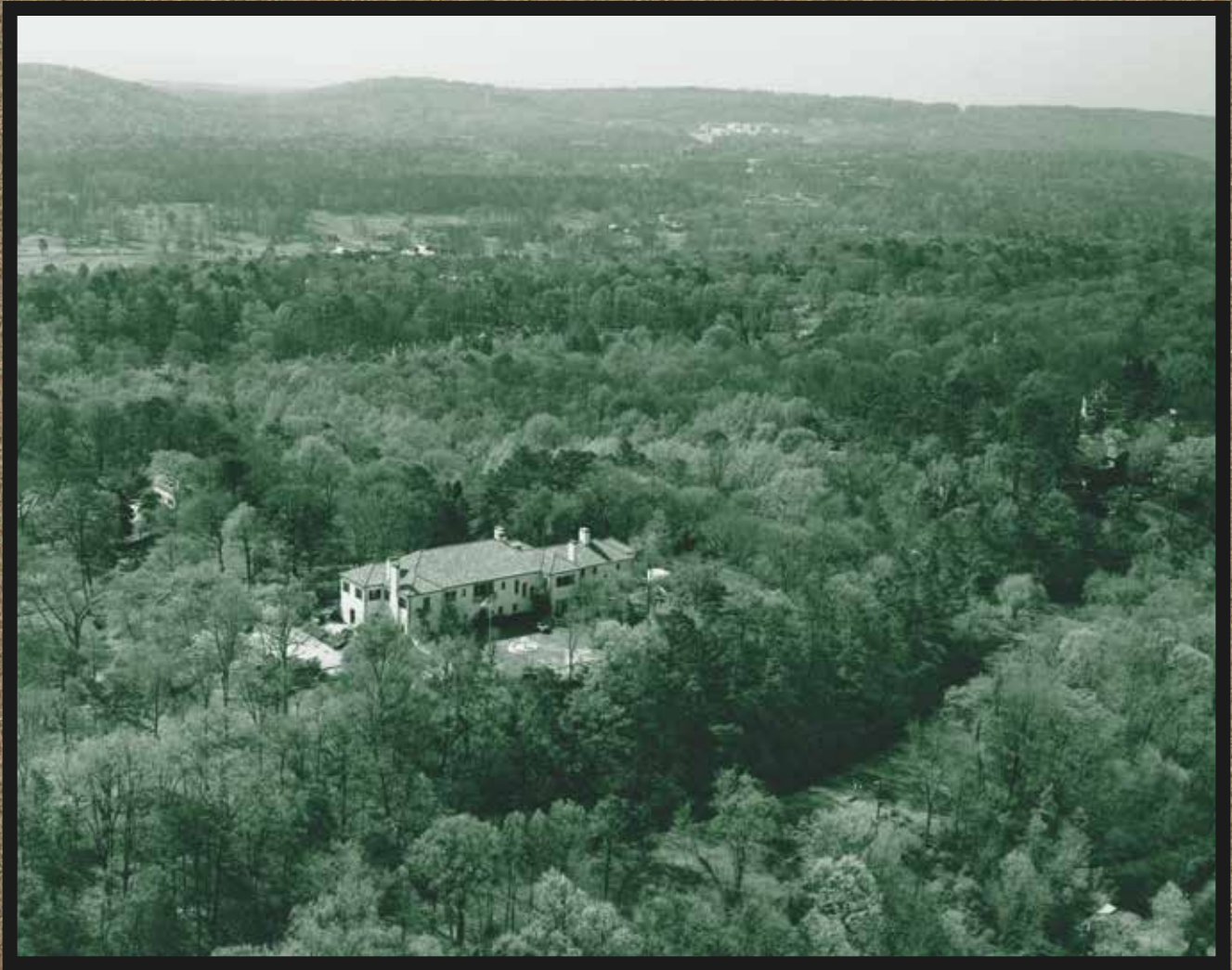
Woodward Estate, with Altamont Parkway and Altamont Park, below , looking south to Shades Mountain. Jet Lowe, Historic American Engineering Record AL-140, 1993.
