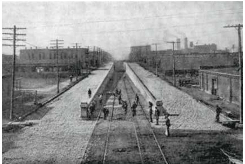
Completed Track Depression, Looking West from East End at 24th Street.
