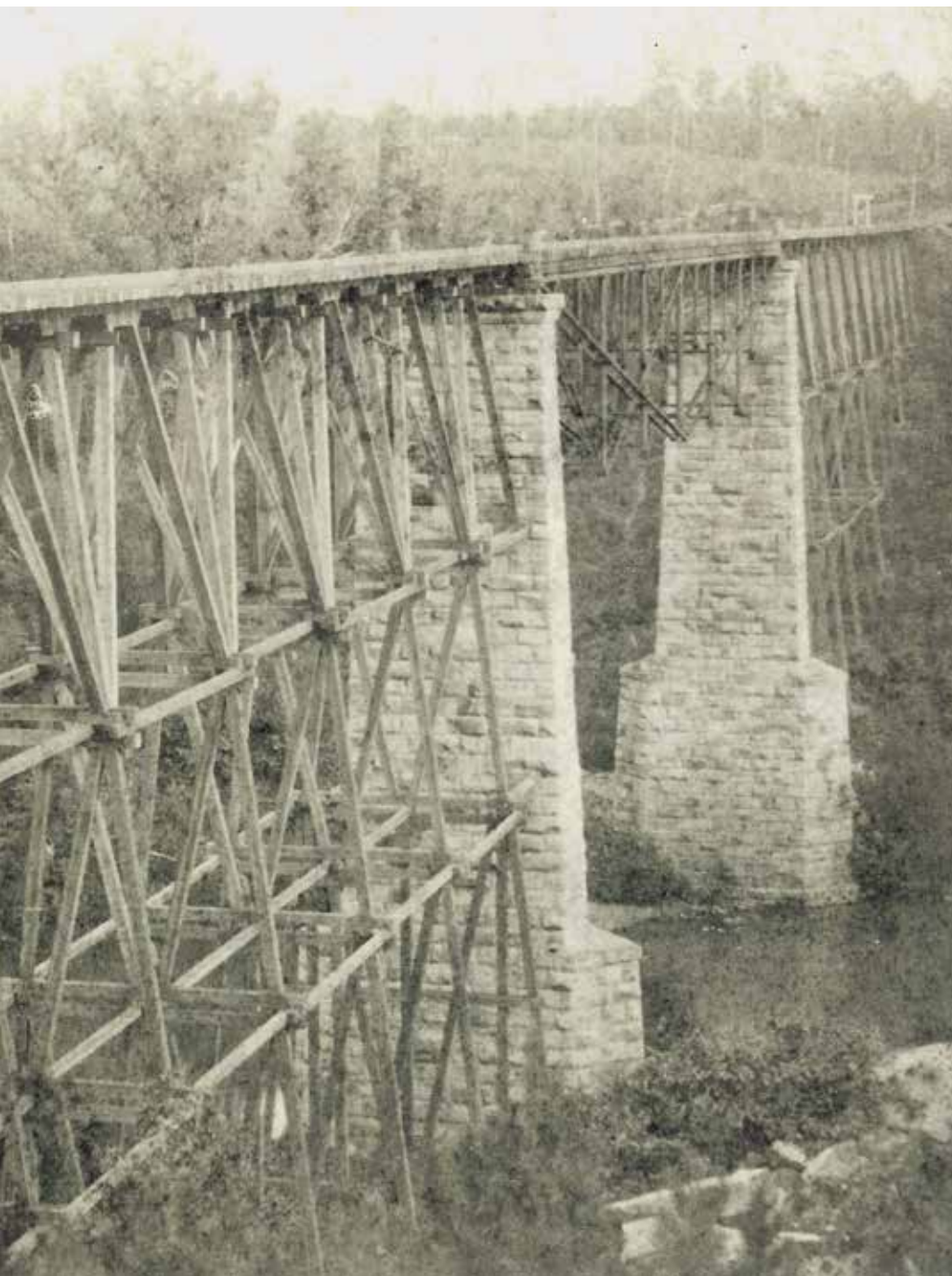
South & North Alabama Railroad Trestle at Warrior, Alabama, 1870s. Courtesy John Stewart and Jim Bennett. A similar 924' long and 40' high trestle once extended across the sag in Elvira Road as it arrives at today's Brock's Gap Training Center.
