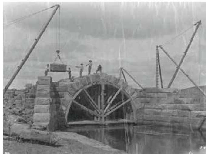
Engineers directing the building of a stone culvert. Dave Rathfon, The Story and History of the 1864 Stone Arch Culvert Railroad Bridge , www.backtobradford.com .
