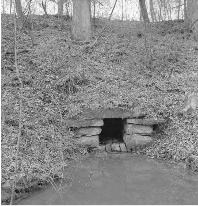
Box culvert, east of the Ross Creek Culvert and similar to the culvert carrying an unnamed tributary under the railroad fill beneath today's Elvira Road, Jet Lowe, 2017.
